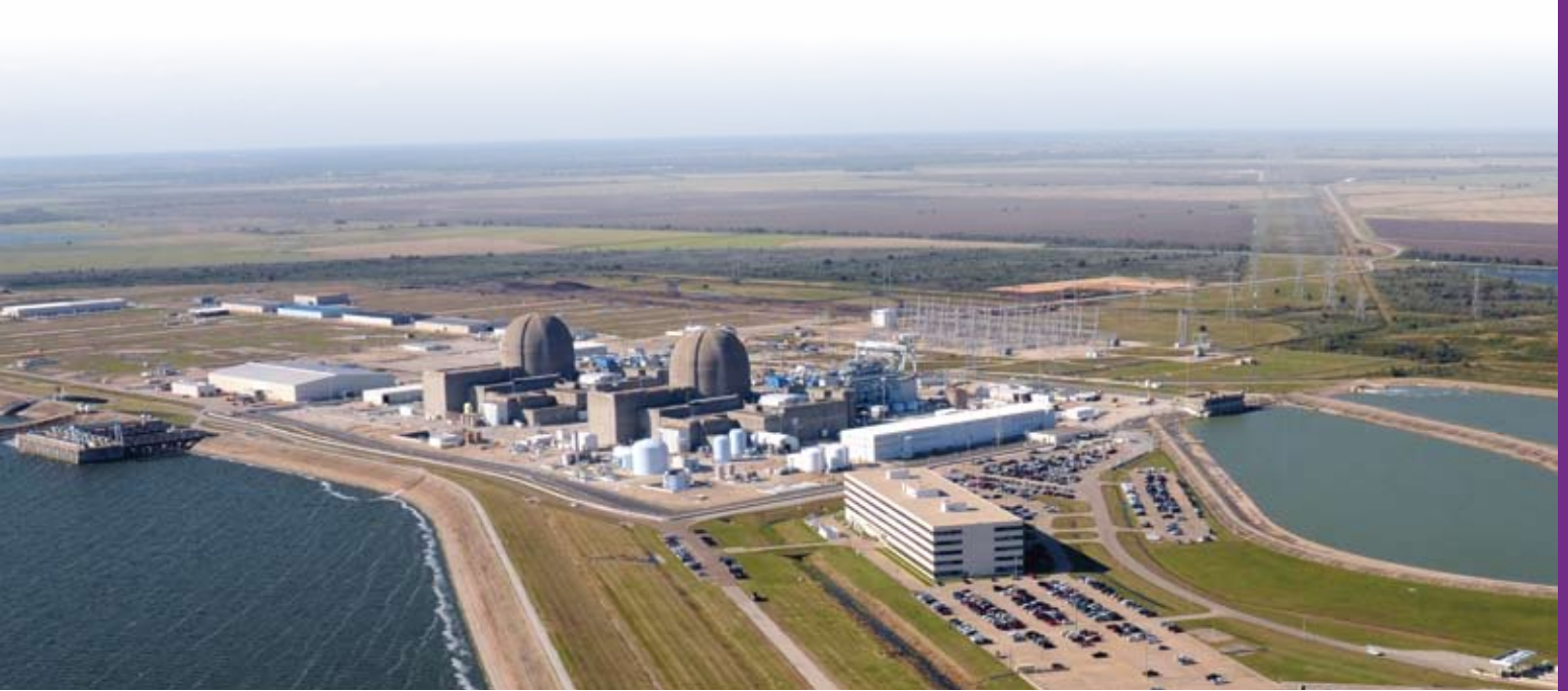
Photo courtesy of South Texas Project Nuclear Plant near Bay City
